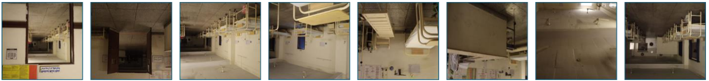
Figure 2 Various views of the male medical ward at Jinnah Memorial Hospital, highlighting entry points, patient and attendant facilities, lighting conditions, ventilation issues, and staff areas that need improvement to enhance patient comfort and care quality.
